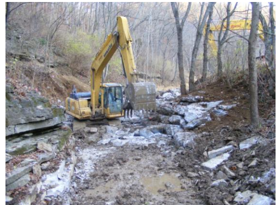
During: construction of rock structures.
