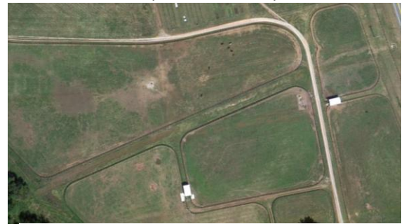
Exclusion fencing and drainage swale, 2010.
