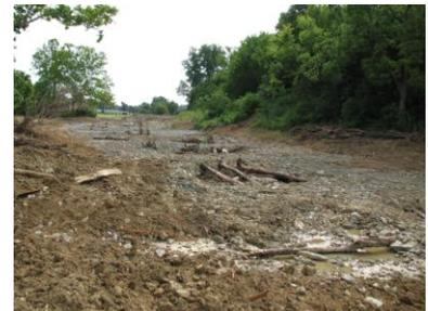
*Floodplain excavated, pools and riffles created & wood installed.*
