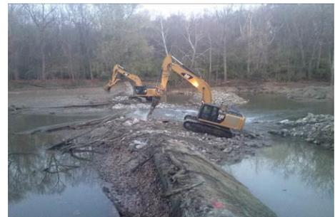
*Excavators removing 300' wide dam.*
