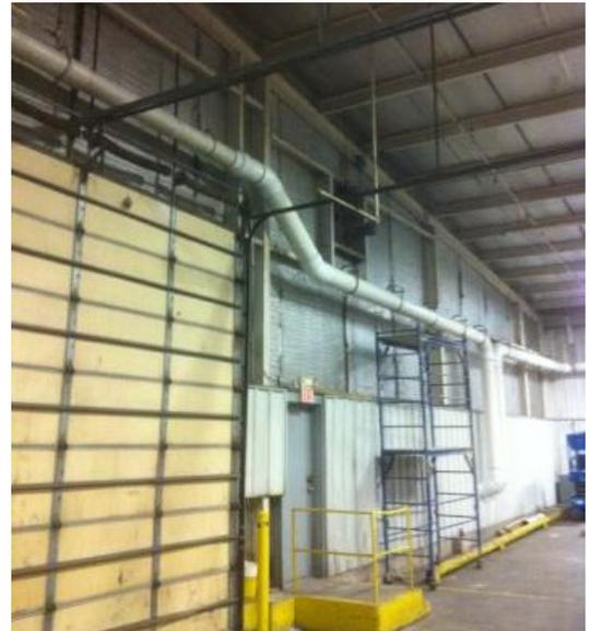
New roof drain lines from internal roof gutters increased capacity and prevents flooding in the building.
