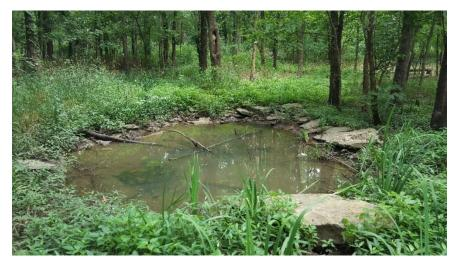
In June, 2019, EcoGro returned to the park to stabilize eroded banks around the blue hole. This was accomplished by removing soil and creating a more shallow and stable slope. Excavated soil was used to redirect flows of runoff from adjacent industrial properties. This work was followed by the installation of native wildflowers by volunteers. As a result, the water of the blue hole is cleaner and clearer.
