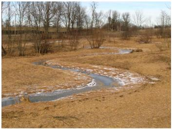
natural fit. Not only did the use of onsite materials provide the most realistic appearance, but also authentically represented the creek's natural form. Many trees and shrubs removed during excavation were stored onsite and transplanted after the final grade was established.
